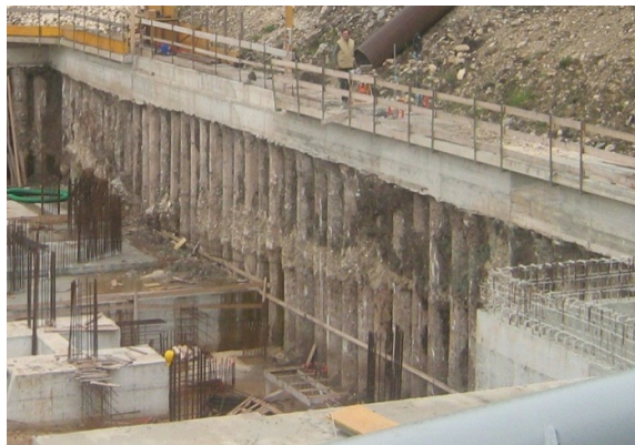
Figure 1. View of the northern part of the wall
