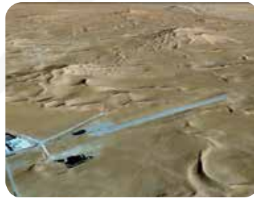
Berkine airport - Algeria
