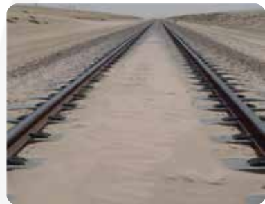
Ballast contamination
