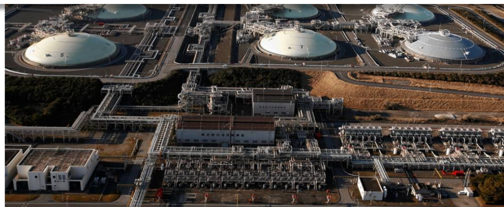
LNG storage tanks near Tokyo. Low natural-gas prices have blunted Japan's push into renewables. PHOTO: ISSEI KATO/REUTERS
