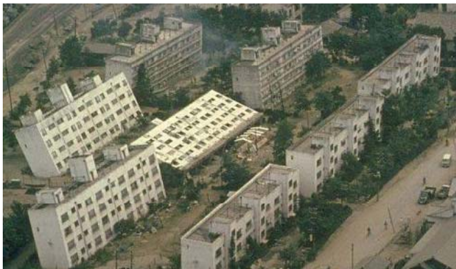
1964 Niigata (Japan) earthquake
